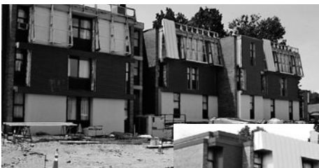
Right: After roof additions and mansard roof panels
