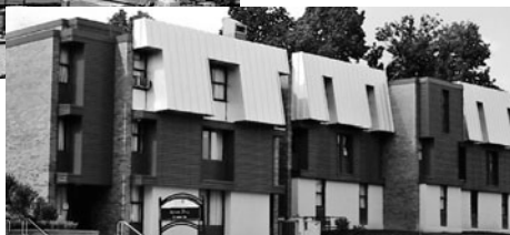
Left: Before construction
